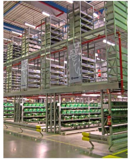
With Multi-tier Pallet Racking from Constructor, you can create manual pick-lanes for your teams at various levels, by providing walkways built into the pallet racking structure.
